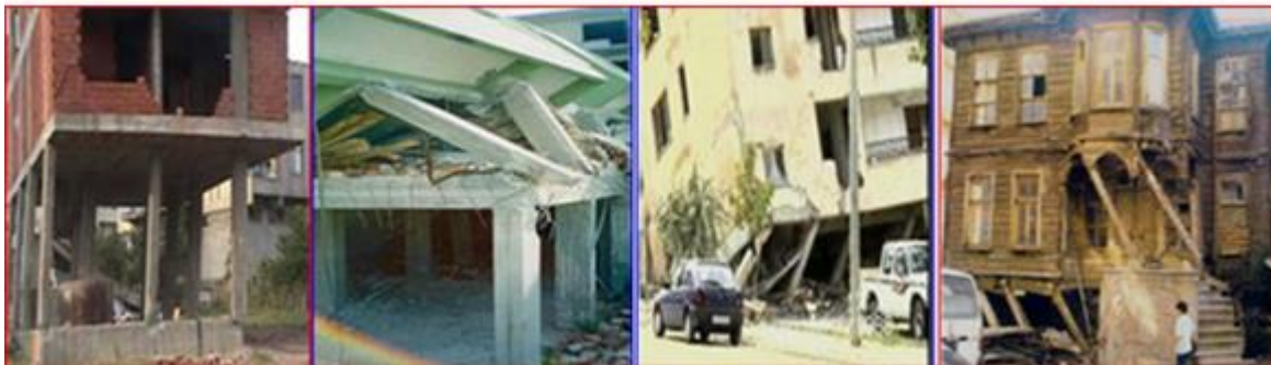
Fig (15) weak story failure (Nevzat Kirac, 2011)
