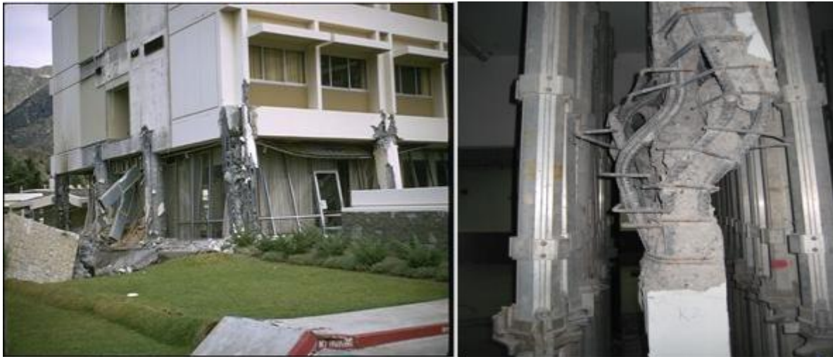
(FIG(54) failure in column due to discontinuity in lateral resisting force San Fernando- California-USA) (Mahin, 1991)
