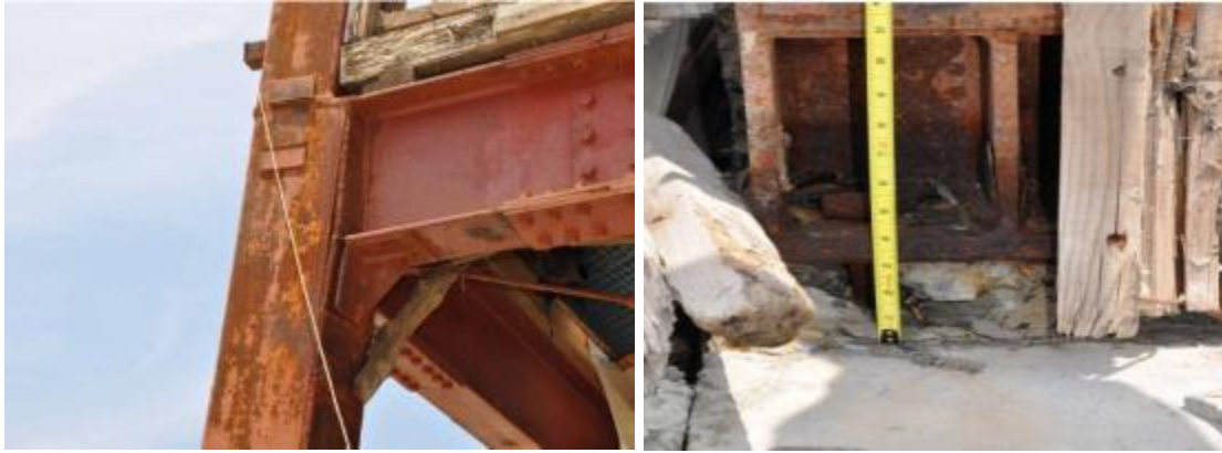
Fig (65) weld failure due to excessive inter-story (James M. Ricles, 2011) base plate detached due to excessive interstory drift (James M. Ricles, 2011)
