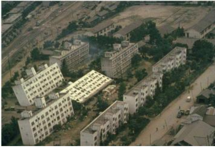
l FIG(10) liquefaction failure (Bhattacharya, 2007)
