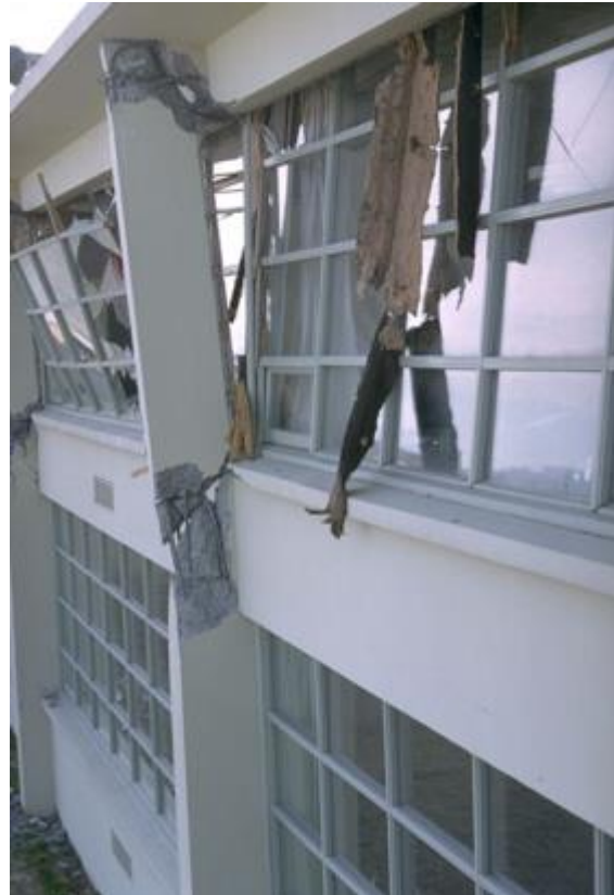
Fig (59) column failure due to poor detailing column (Heidi Faison, 2004)
