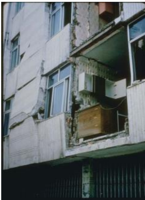
Fig (61) Masonry in filled failure (Earthquake Damage, 1990)
