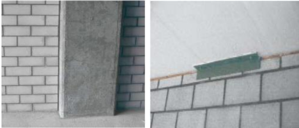
Fig(34) providing joint between frame and infill masonry(Bachmann, 2002)
