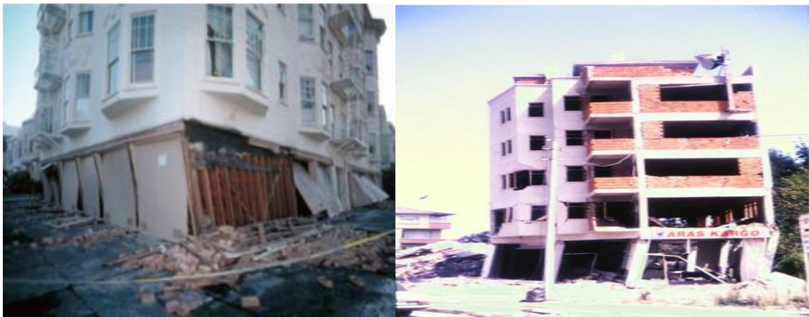
Fig (55) soft storey failure in Loma Prieta earthquake damage in San Francisco (Braile, 2003) and in Turkey (Polat Gulkan, 2002)
