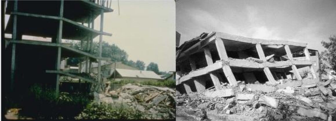
Fig (62) beam failure due to excessive plastic hinge occurrence (NOAA, 1990)
