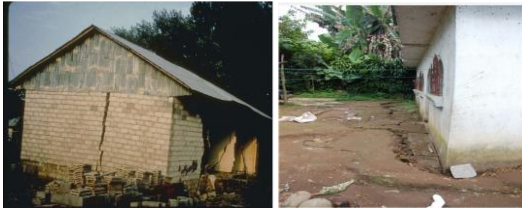
Fig (6) foundation settlement (Damage, 1990) foundation settlement foundation settlement (EERI, 2011a)
