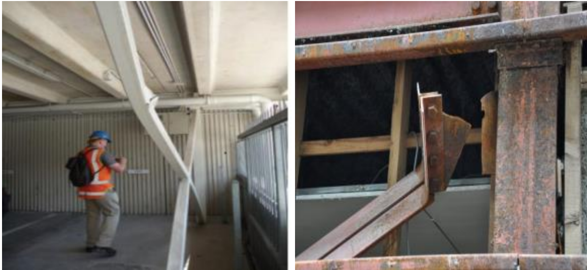
Fig (67) bracing failure due to insufficient section (Clifton, 2011) (James M. Ricles, 2011)
