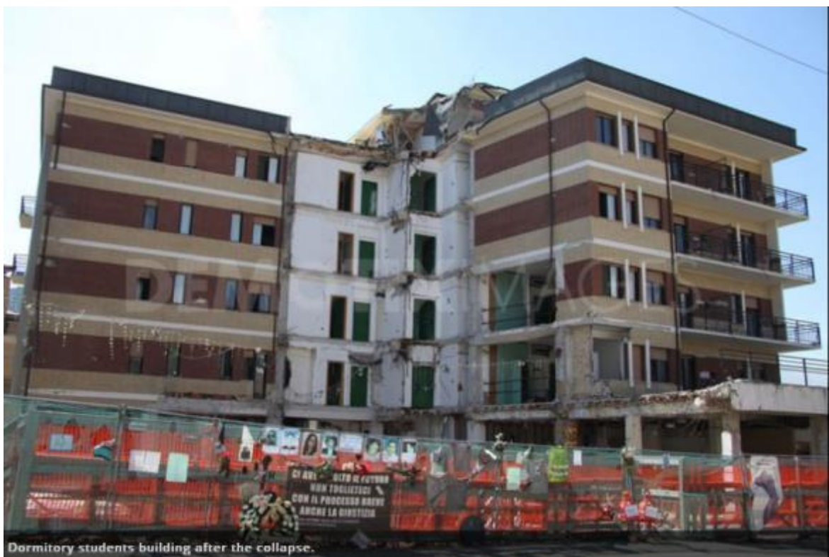
Fig (56) re-entrant corner failure in Aquila, Italy (albani, 2012)
