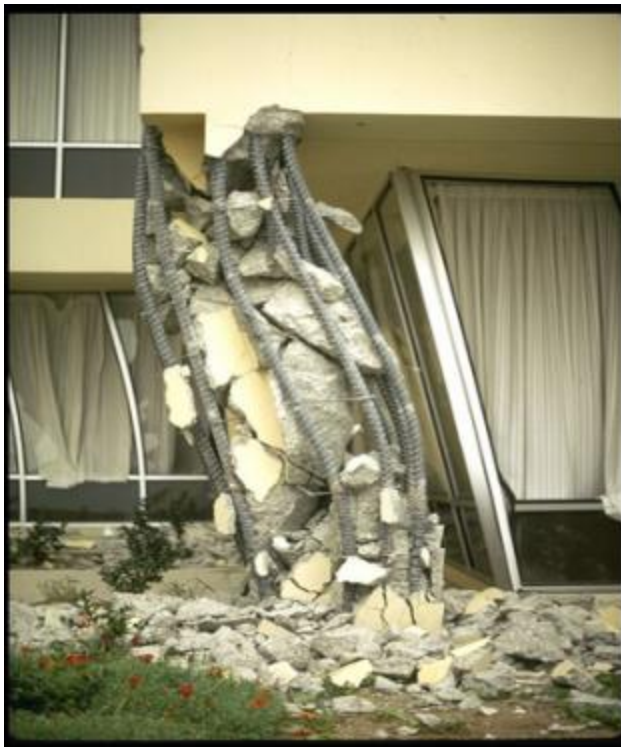
Fig (59) column failure due to poor detailing column (Heidi Faison, 2004)
