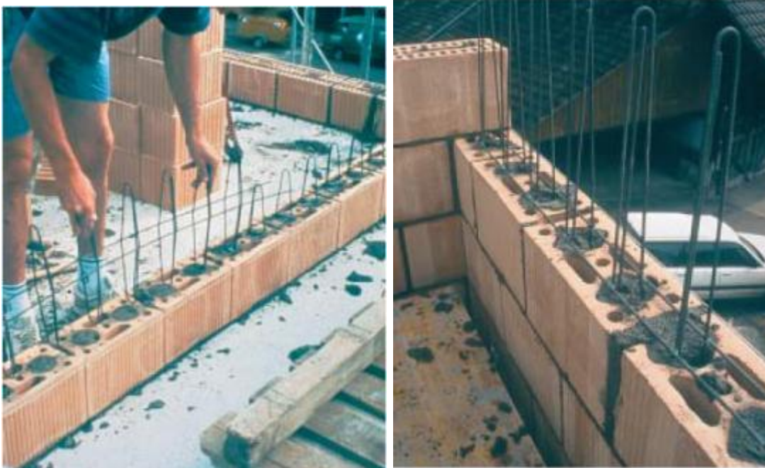
Fig (33) improve the masonry wall against earthquake loading (Bachmann, 2002)
