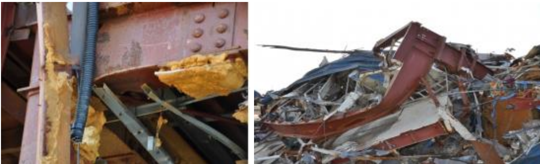
Fig (64) beam failure due to excessive plastic hinge occurrence (James M. Ricles, 2011)
