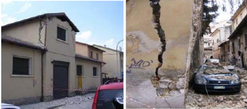
Fig (60) out-of-plat failure (unipv, 2013)
