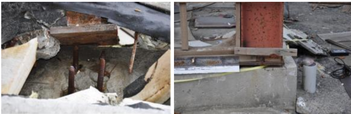
Fig (66) overturning failure caused base plate rapture (James M. Ricles, 2011)
