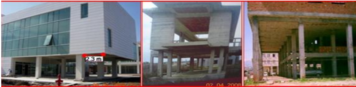
Fig (14) weak story before earthquake (Nevzat Kirac, 2011)
