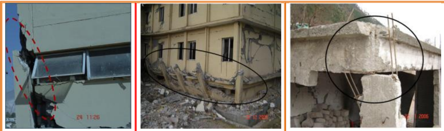
Fig (21) failure due to poor detailed reinforcement and poor construction (Y B Marhatta, 2007)
