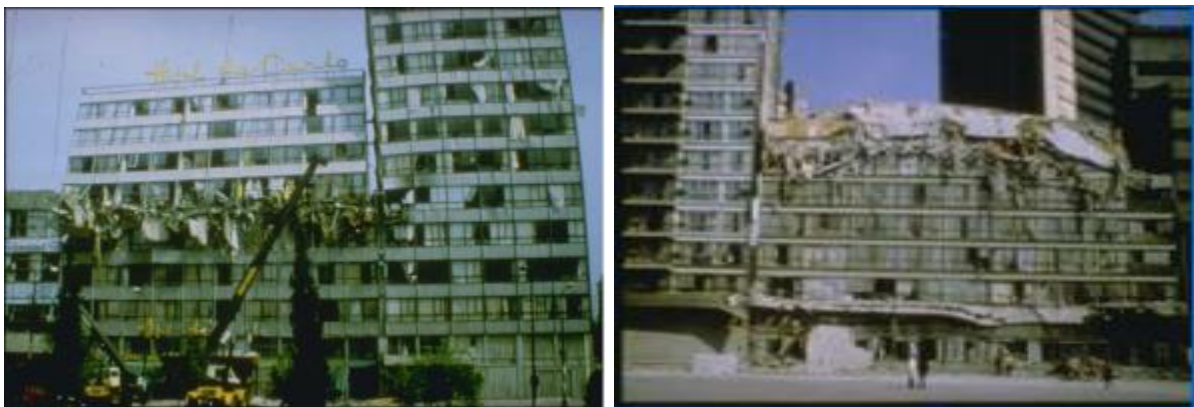
Fig (58) pounding failure Maxico-city (Index)
