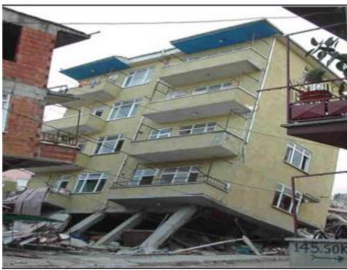
Fig (11) soft story failure (Alarcon, 2009)
