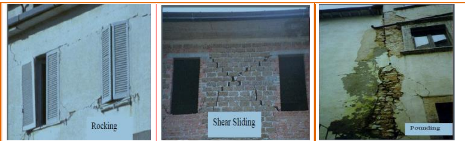
Fig(22) failure modes in masonry (Rocking, shear sliding and Pounding )(Rush, 2007)
