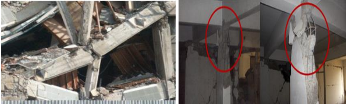
Fig (57) weak column strong beam failure in Banda Aceh, Indonesia (Ahmed Ghobaraha, 2006) and in Pakistan (Yasir Irfan Badrashi, 2010)
