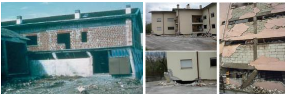
Fig (23) failure in column due to partially infill masonry(Bachmann, 2002, G. Uva, 2012)
